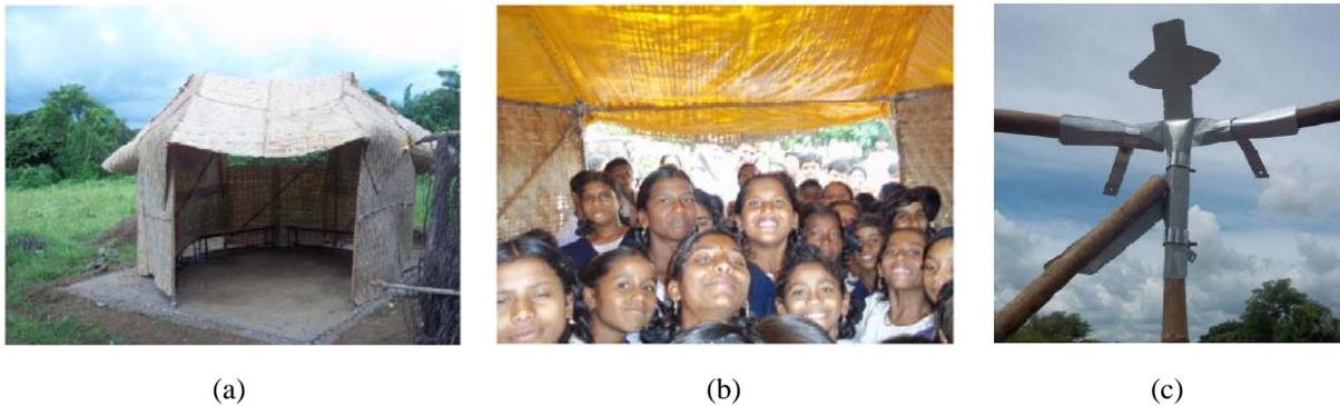
Figure 3: (a) bamboo hut in Pabal, summer 2010; (b) School pupils in the hut; (c) Detail of the 5-point metal plate connection
